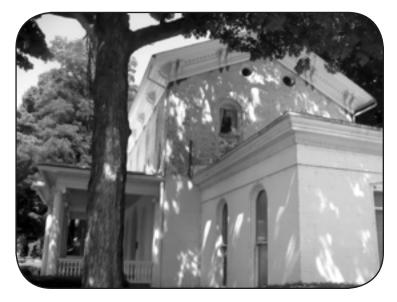
Two portal windows, hidden for over fifty years by aluminum siding, were revealed during the recent siding removal. The original brick is in good condition, although tuck pointing will be required.
